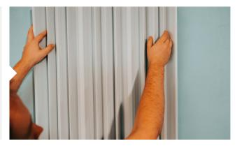
Depending on the condition of the wall, it is recommended to apply a thicker line of glue by enlarging the nozzle of the cartridge using a utility knife.
